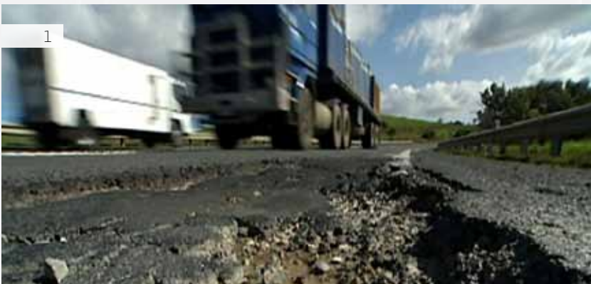
1. Upgrade works to the Midland Highway are on track to begin this year
